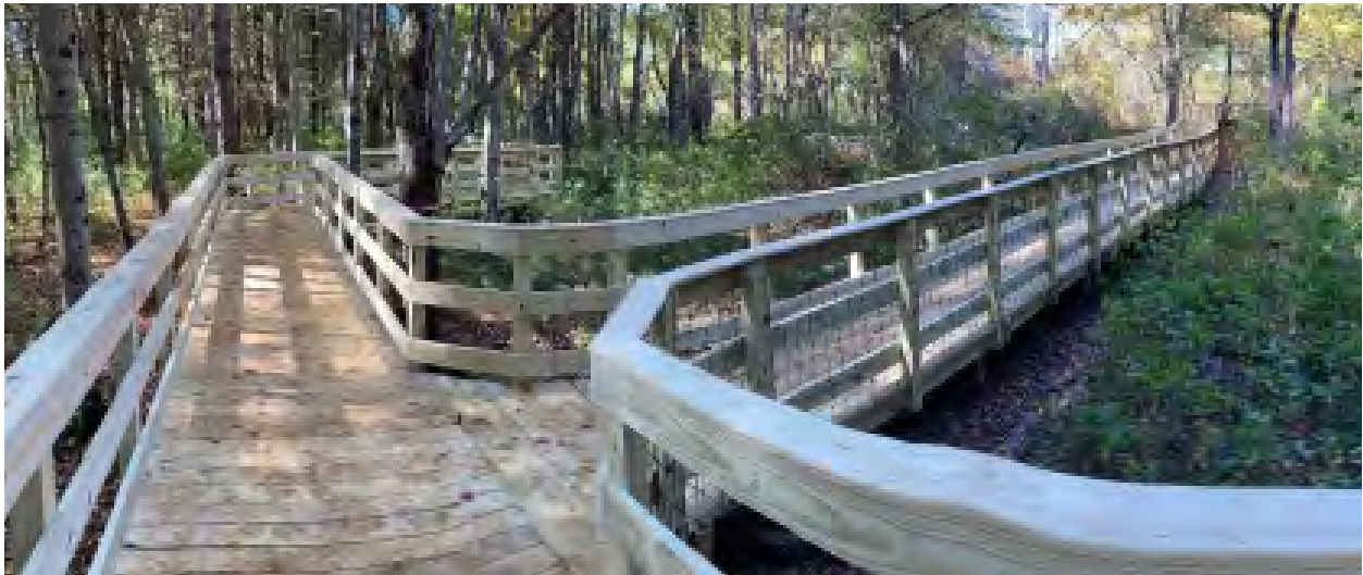
Newbury Court Boardwalk, Concord, MA
